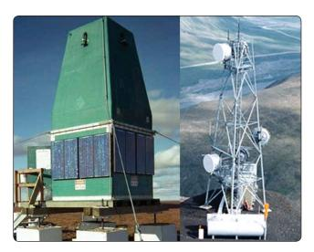
Figure 11-135. Low power requirements allow remote ADS-B stations with only solar or propane support. This is not possible with ground radar due to high power demands which inhibit remote area radar coverage for air traffic purposes.
